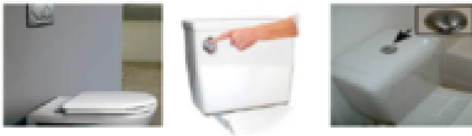
Photographs: Low flush cisterns
